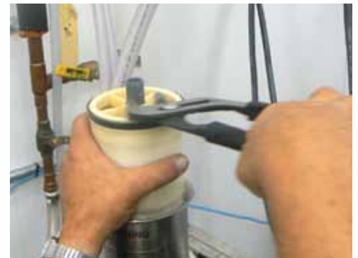
Once the filter is loose, pull it all the way out and discard.
