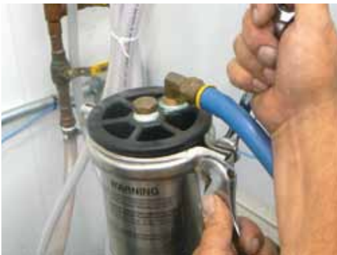
Now you need to change the filter in your Membrane. Use 2 wrenches to loosen the nuts on the collar.
