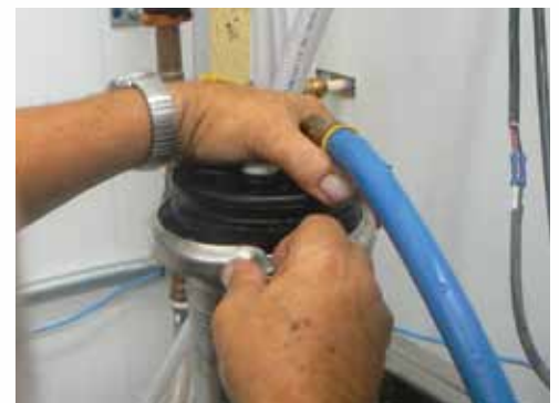
Push the cap down until it seats itself. Then put the collar back on. Turn water and power back on.
