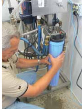
Unscrew the PreFilter counter clockwise until it comes off. You may need to use a wrench or hammer to get it started.
